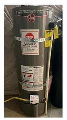
If installed in a garage, residential equipment or appliances which have an open flame or electrical components that may produce a spark, must be raised up, locating the ignition source at least 18" off the floor. There is an exception where the appliance is flammable-vapor-ignition-resistant (FVIR), a feature provided typically on all residential water heaters, starting back in 2004.
